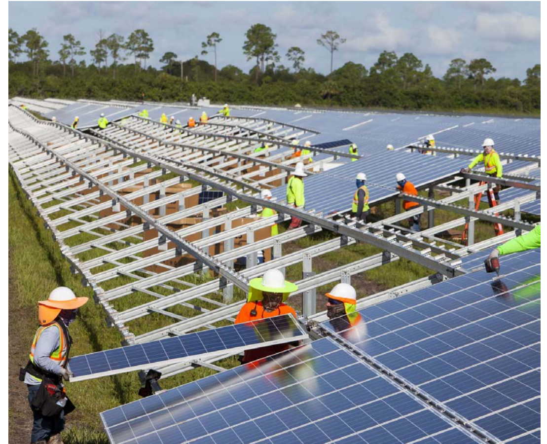
Workers install solar in Florida Photo: Google Images
